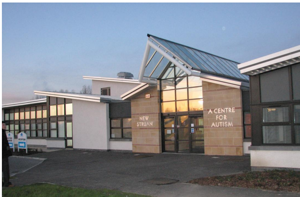
Figura 13 - Centro New Struan School
