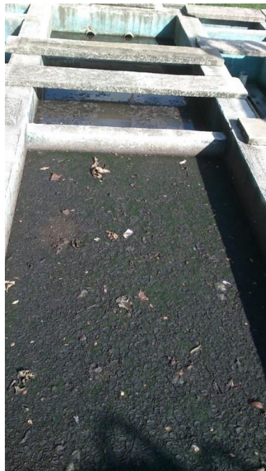
Figura 2.2. Decanto digestor
