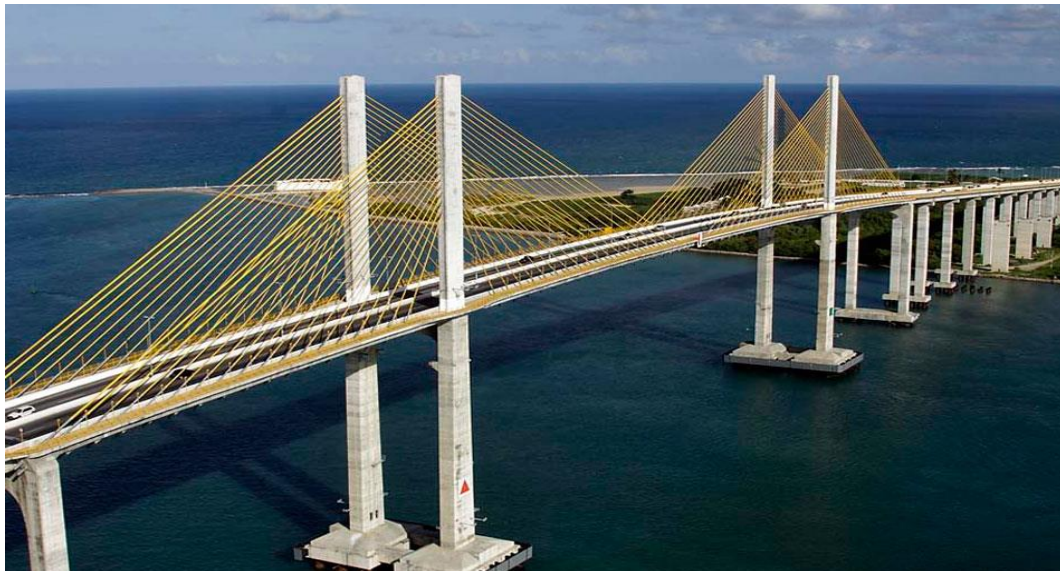
Figura 01 – Ponte Newton Navarro, Natal (RN)
